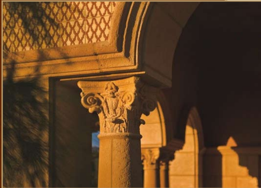
DETAIL, HAND CUT STONE WORK
